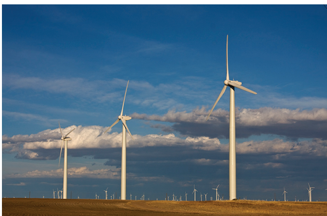
Wind farms such as this one near Grover, Colorado, can include more than 200 turbines.
